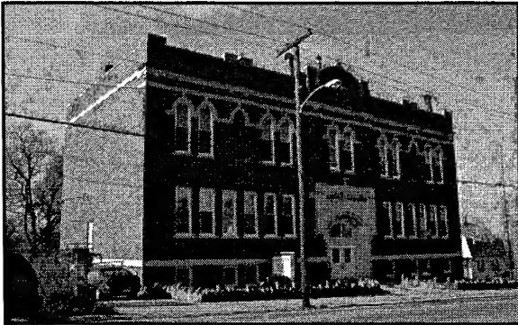
Cross Evangelical Lutheran School Building at 2902 South 20th Street (DO09:0110-010)
